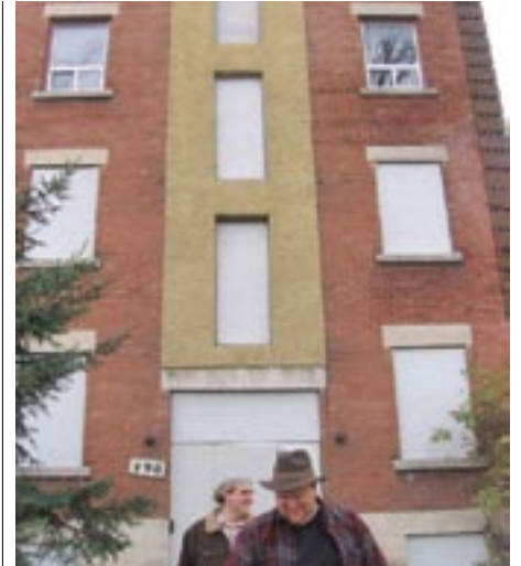
Chiara House at 490 Maryland St., Winnipeg, is a century-old apartment building that needs significant renovation to "turn it into affordable housing that includes relationships in the community," says Jamie Arpin-Ricci, pastor of Little Flowers Community, a church plant of Mennonite Church Manitoba.
