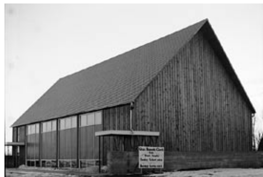
Grace Mennonite Church, Winkler, Man., first met as an English-language congregation at Winkler Bible School. This facility was built in 1962.
