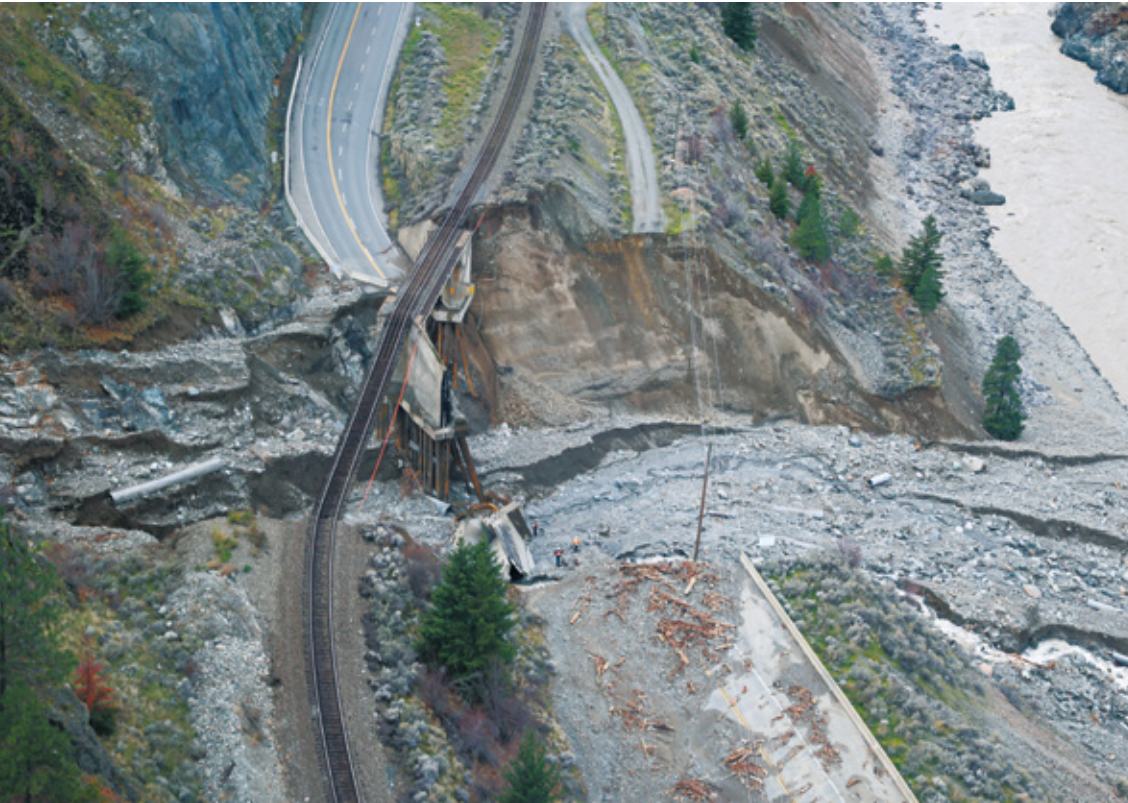
B.C. MINISTRY OF TRANSPORTATION AND INFRASTRUCTURE PHOTO (CC BY-NC-ND 2.0)
